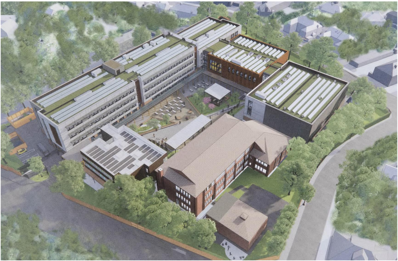
Above Aerial View
